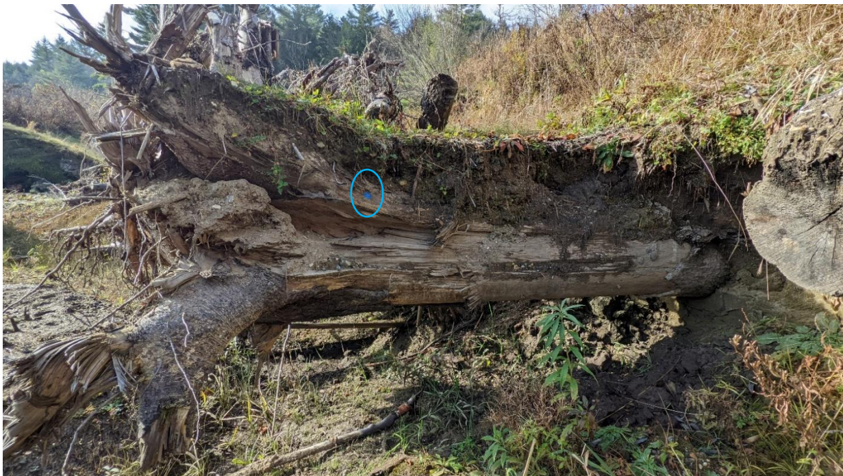
Figure 4. Image of an installed rootwad at WR2 with the blue metal tag highlighted with a blue circle.
