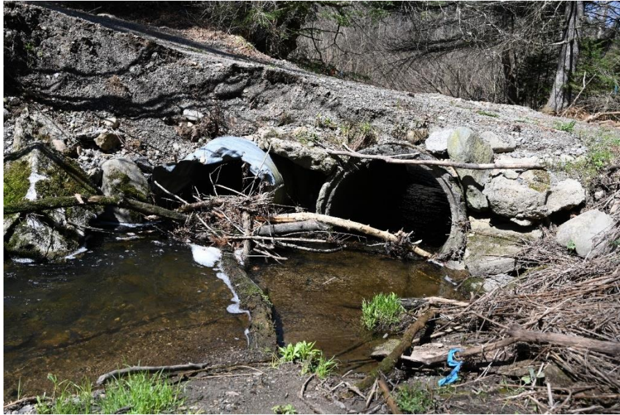
Figure 68. View southwest of the inlet side of the culvert that carries Trout Brook under the west access road.
