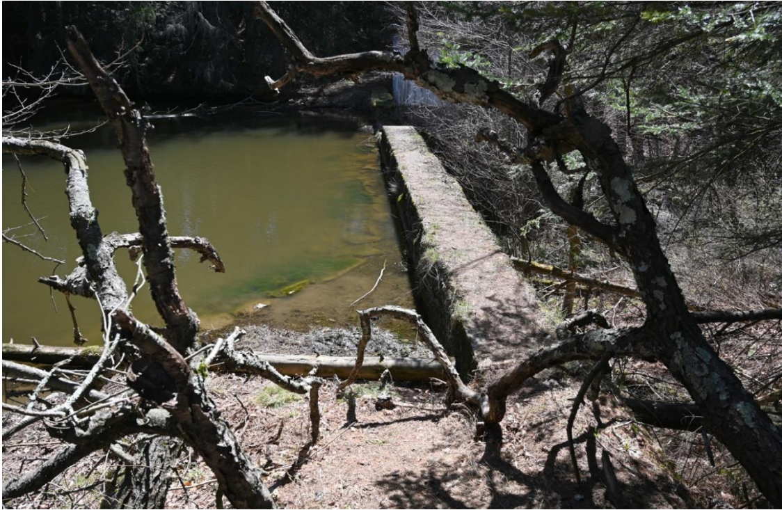
Figure 57. View of the upstream stone pavement feature, looking eastwards.
