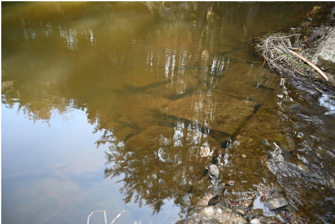
Figure 58. View of the pavement feature on the upstream side of the dam, looking northeast.
