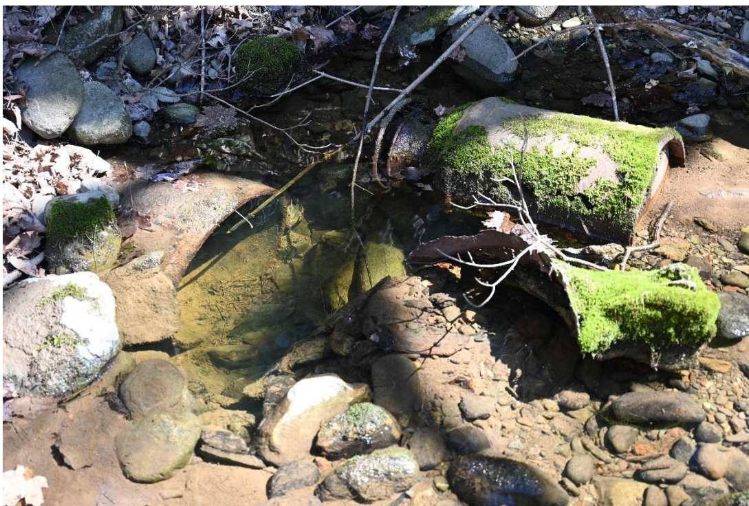
Figure 54. View of iron pipe / possible “blow-off pipe” south of the gate house and control chamber on the left side of the spillway.
