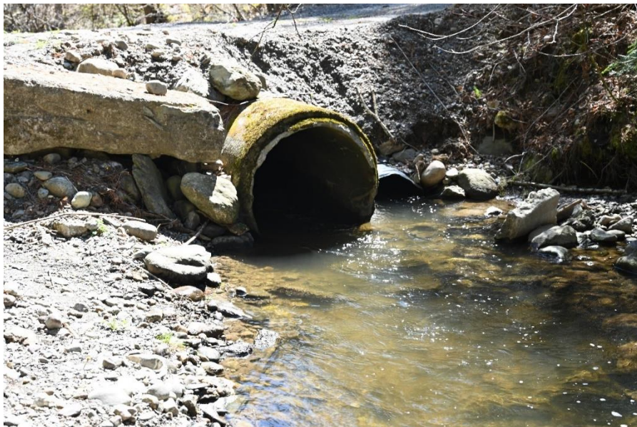
Figure 69. View southeast of the outlet side of the culvert that carries Trout Brook under the west access road.
