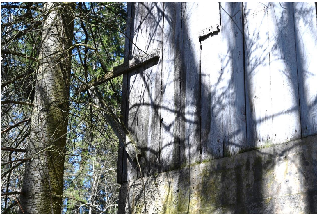
Figure 53. Close up view of bracket on back of gate house structure.
