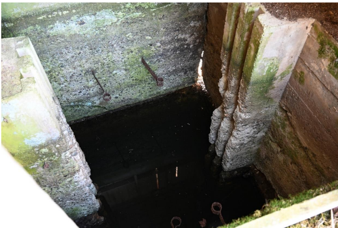
Figure 50. View of the interior of the gate chamber; note the concrete formed guides for the copper screens and the metal gate thread guides.
