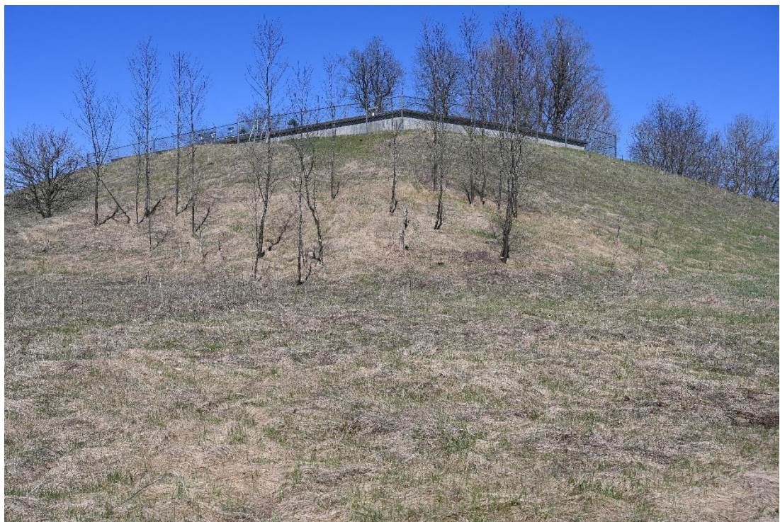
Figure 67. View northeast of the Concrete Reservoir.
