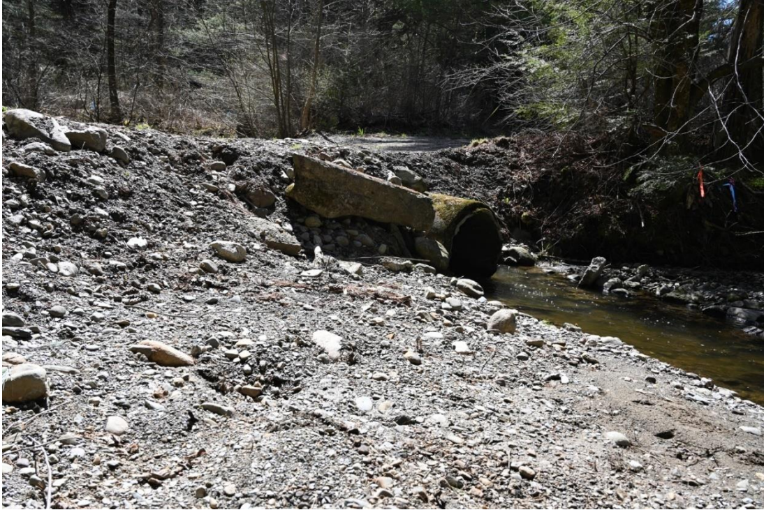
Figure 17. View of a cement culvert on Trout Brook and an extensive area of fill around it on the proposed western access route, looking southeast.
