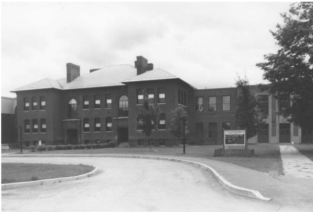
Figure 97. View southeast of school along the north side of School Street (1984).
