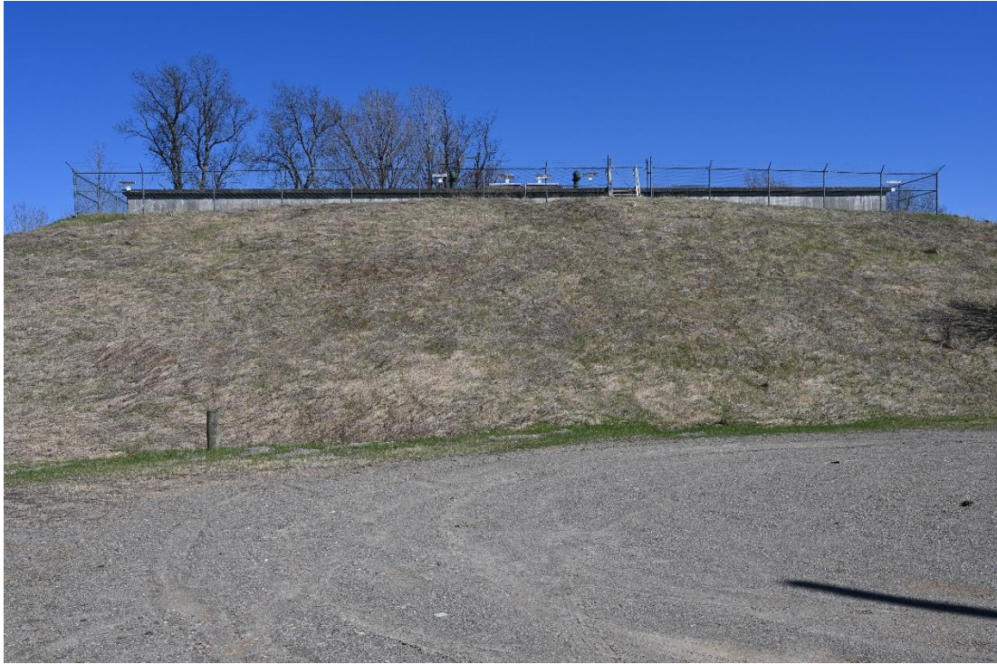
Figure 66. View east of the Concrete Reservoir.
