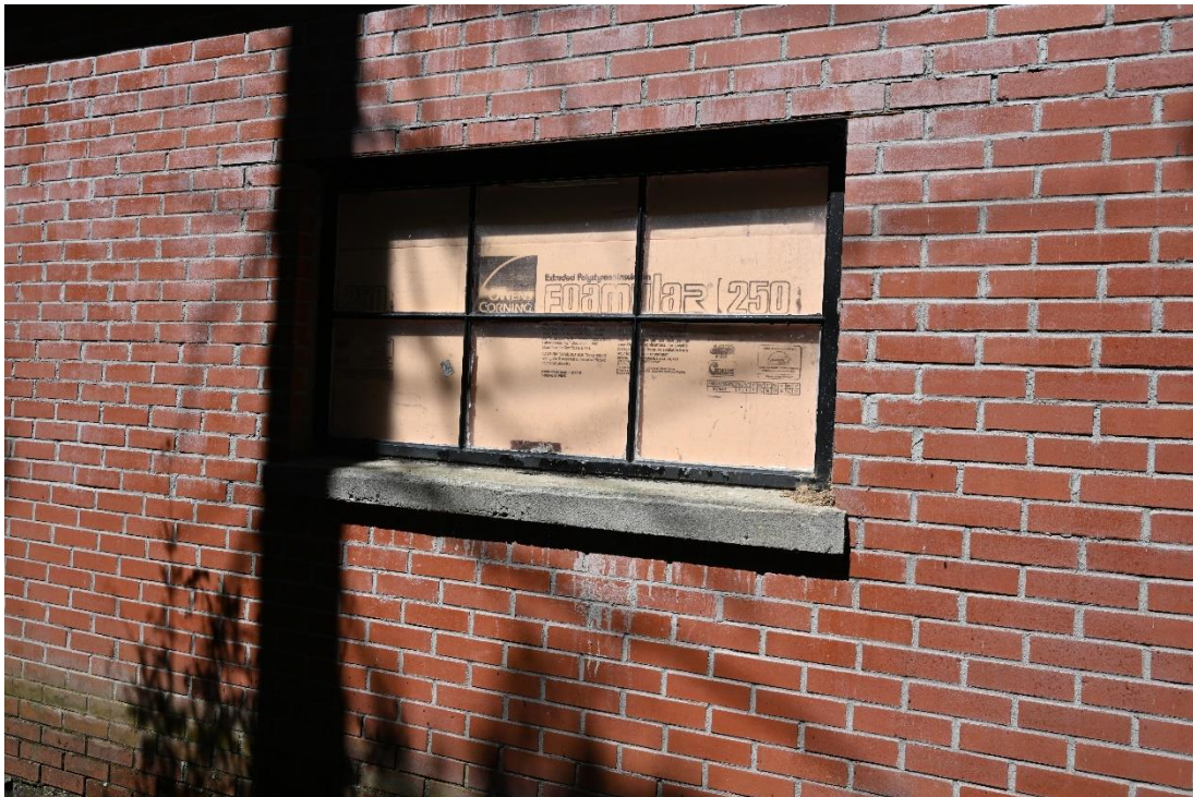
Figure 63. View southwest of window in the rear side of Well House #2.
