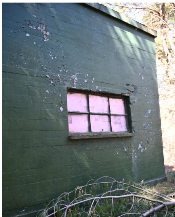
Figure 61. View northwest of the rear side of Well House #1.
