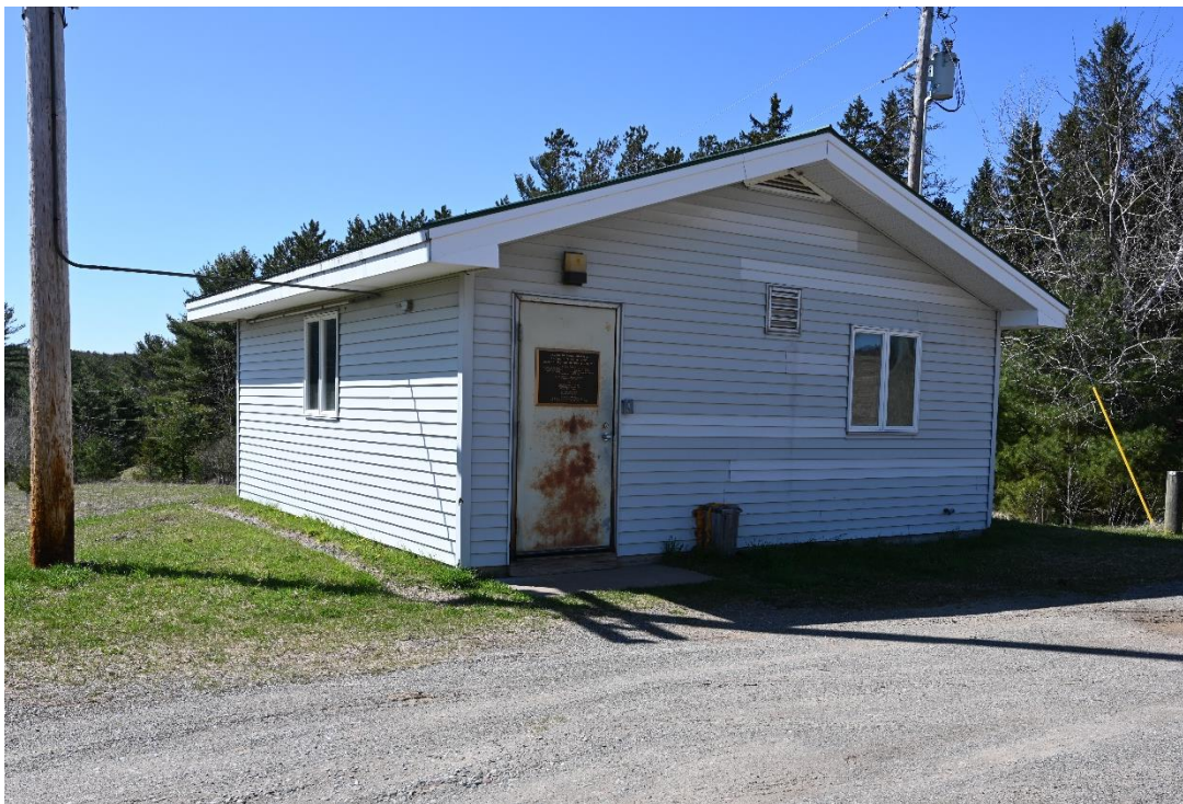
Figure 64. View northwest of the Chemical Feed Building.
