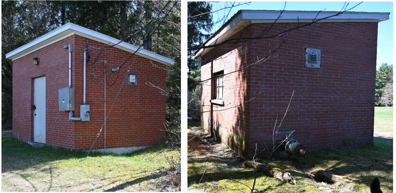
Figure 62. View northeast (left) and southwest (right) of Well House #2.
