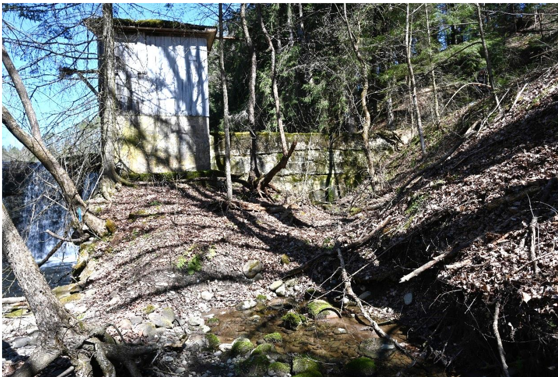
Figure 52. View of the gate house and control chamber on the left side of the spillway, looking west, note bracket on back of structure and pipe to left of milk can.
