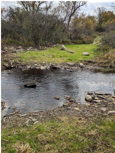
Above: The Dead Creek following bridge removal. The creek is no longer constricted due to encroachment, improving stream flow and water quality.
